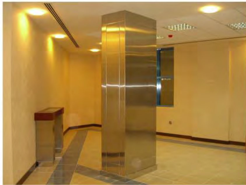
Sheet Cladding Works ▶ Column
