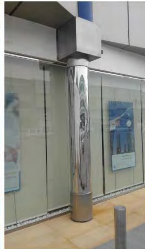
Sheet Cladding Works ▶ Column
