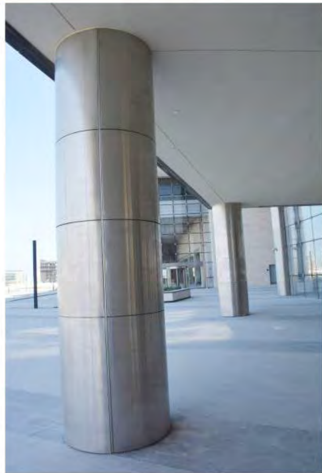
Sheet Cladding Works ▶ Column
